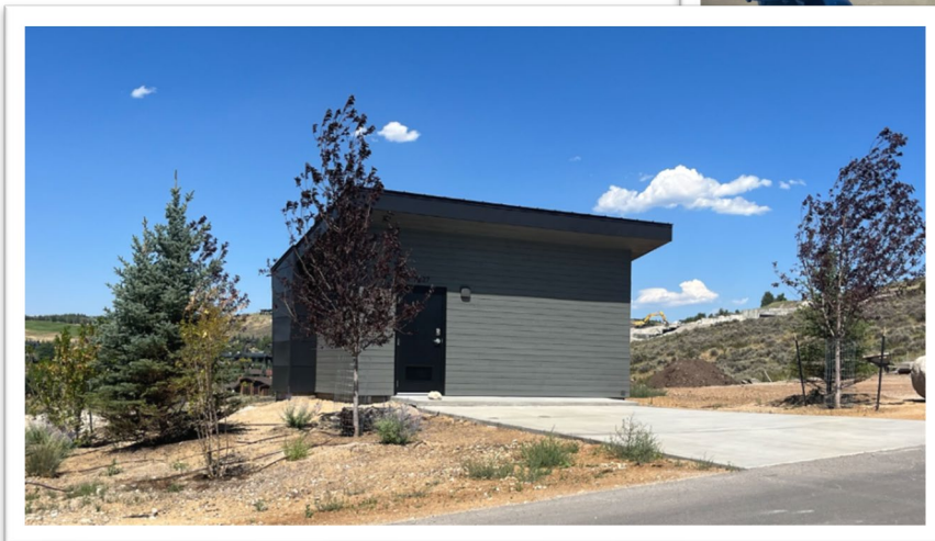
Sage Hills Control Valve Building
