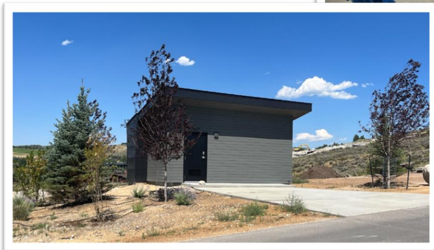
Sage Hills Control Valve Building
