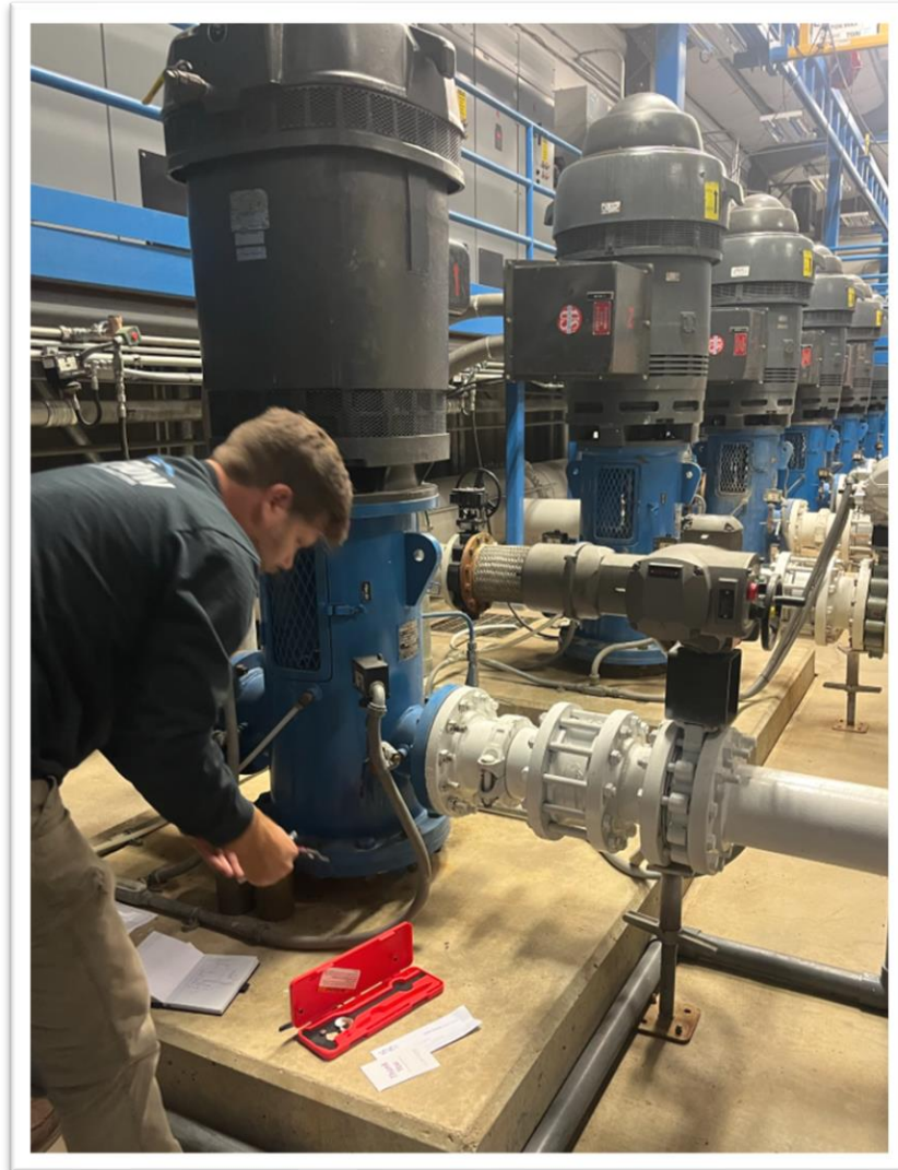
Final Measurements with a Pump Supplier on LC Pump 1
