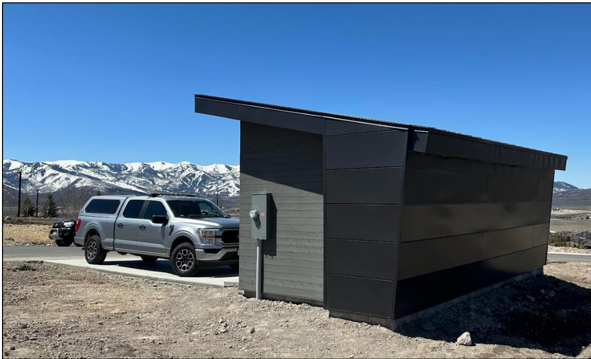
Sage Hills Control Valve Building
