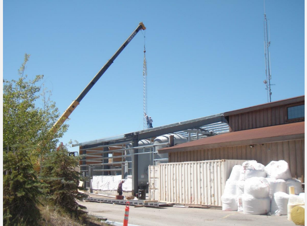
Treatment Plant Expansion Project
